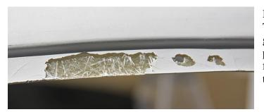
I also have a number of voids and dings to fix. These are right in front where the chin window goes and it will be noticeable. I'm using polyester resin and mixing in chopped fiberglass or glass microspheres, depending on the application.
