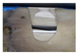
The Mylar will prevent the resin from sticking and give it a nice smooth finish. If I'm lucky it will conform to the existing curved surface and I won't have too much sanding to do.
