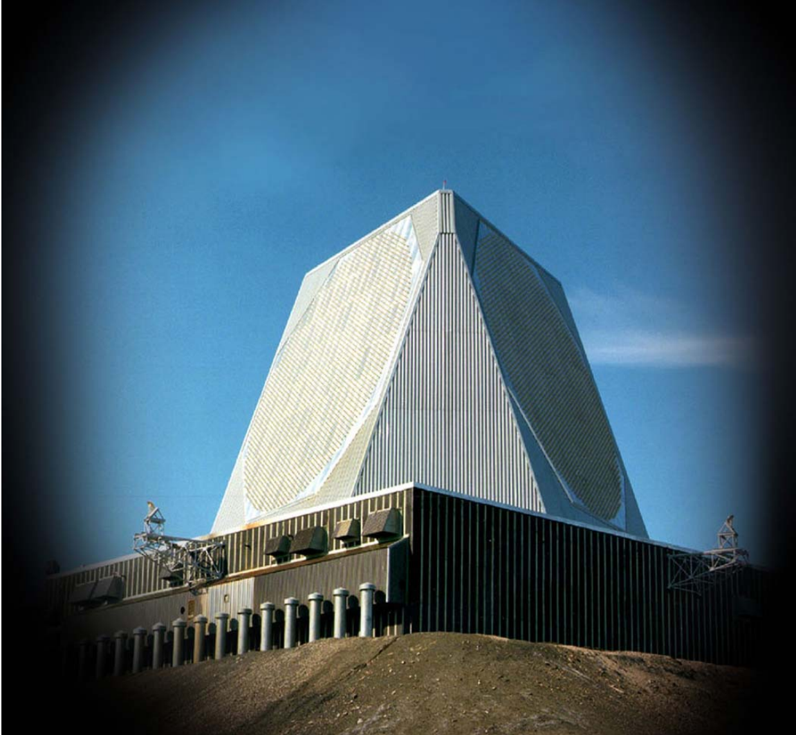
Figure 27-1. AN/FPS-123 PAVE PAWS Radar Antenna 1
